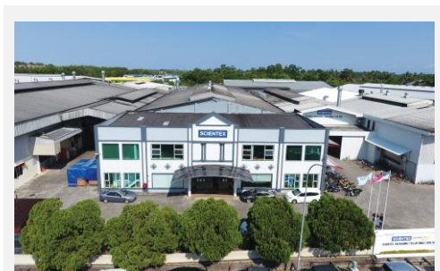
Teluk Emas plant
