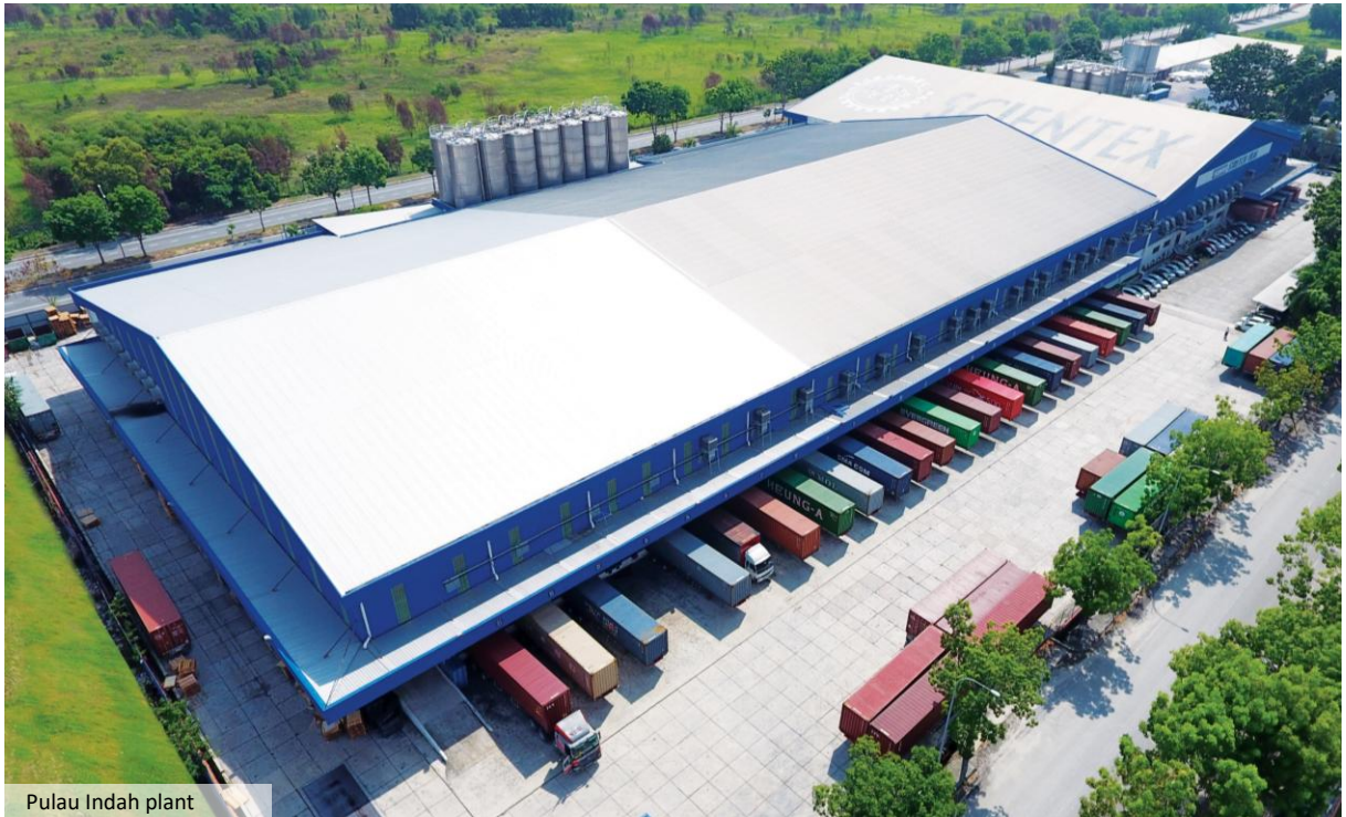
Pulau Indah plant
