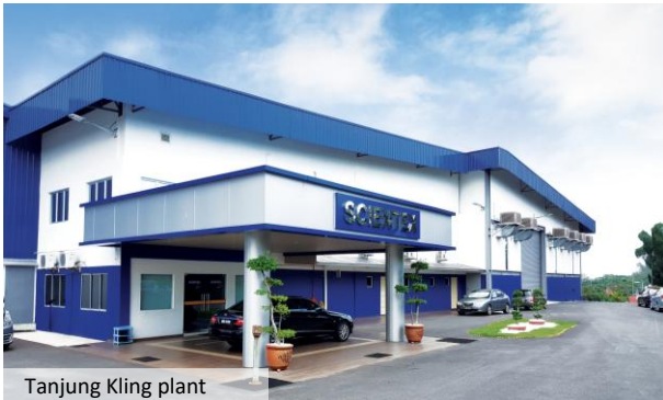
Tanjung Kling plant
