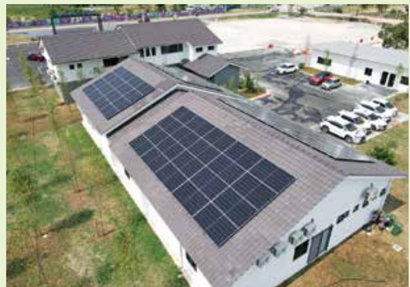
The rooftop solar PV system at our sales gallery
