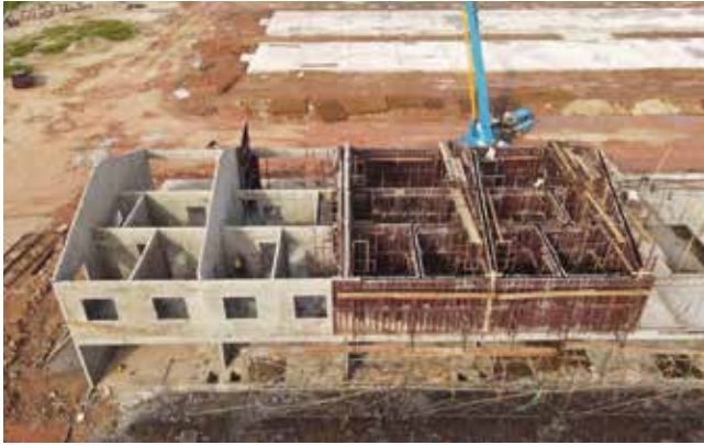
A sample development utilising the IBS construction technique encompasses all wall sections
