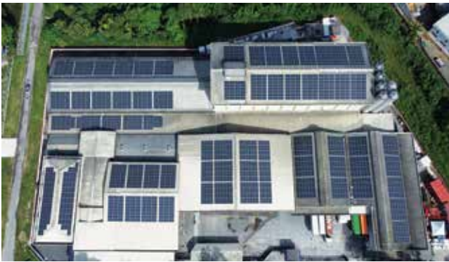
Our maiden solar PV project at one of our manufacturing plants in Ipoh
