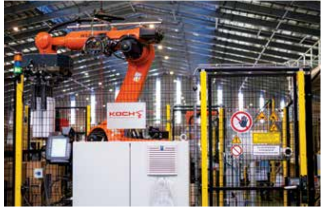
Perimeter safety fence installed at our Robotic Stretch Film Plant in Shah Alam
