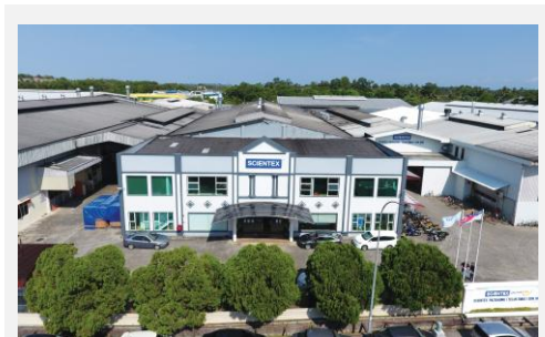
Teluk Emas plant
