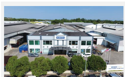
Teluk Emas plant
