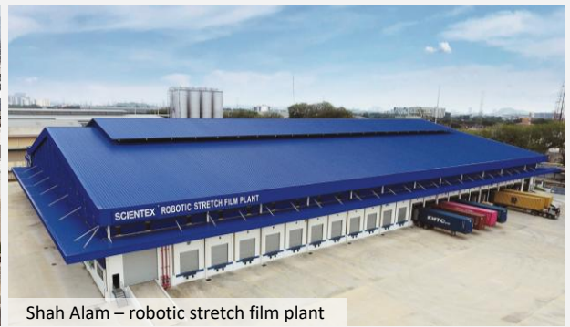
Shah Alam – robotic stretch film plant
