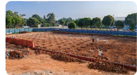
Teluk Emas new warehouse progress
